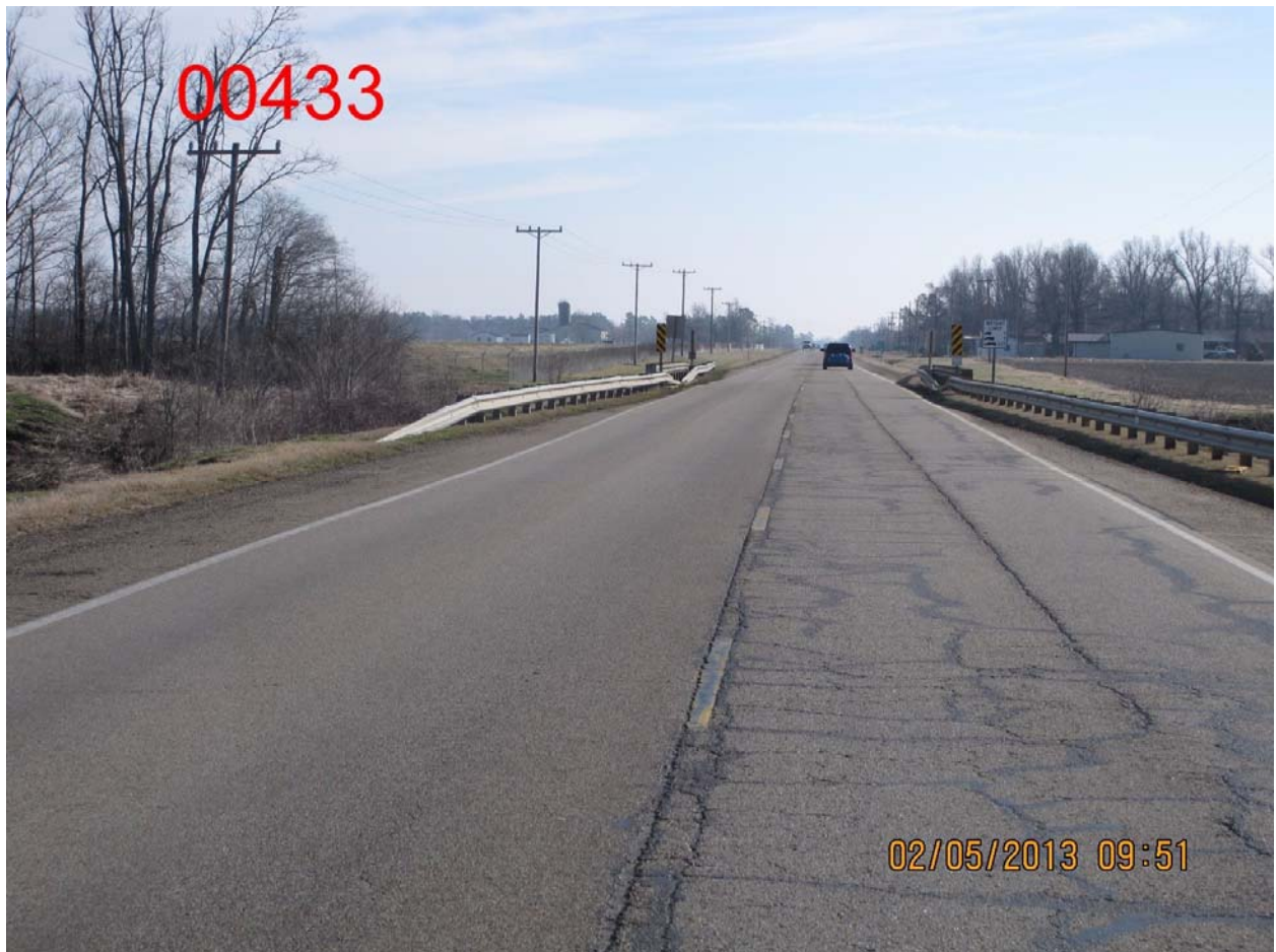
Note: 5 inches of ACHM overlay on bridge deck.
