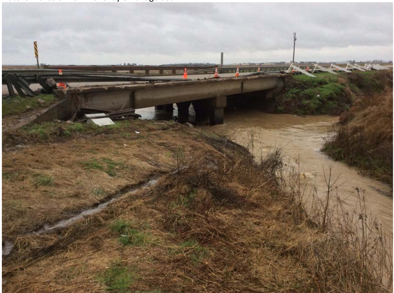
Note: 5 inches of ACHM overlay on bridge deck.
